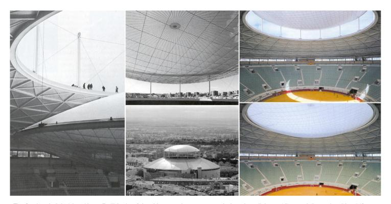
The fixed roof of the Vista Alegre Facilities is a Schwelder-type dome, composed of steel parallels, meridians and diagonals, with a 1/8 rise-span ratio. It is supported on concrete pillars at its perimeter.
